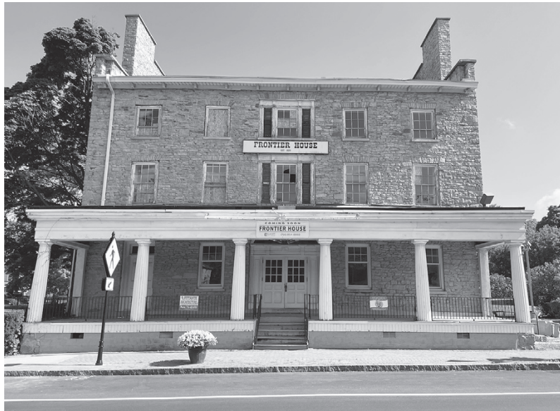
The Frontier House at 460 Center St., Lewiston.
